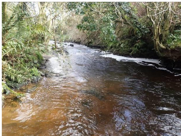
Plate 36 Move instream boulders downstream to main riffle. Clear lateral branches and dead pine on LHS bank. Remove whitethorn trees on LHS bank.
