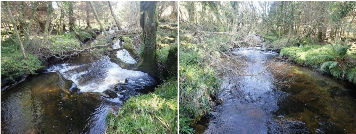
Plate 29 Cut large willow tree trunks and remove fallen branches to expose pool.
