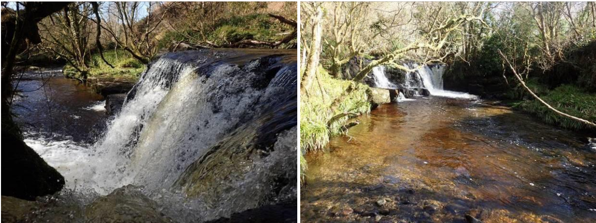
Plate 33 Waterfall and pool (view downstream, left). View upstream (right). Possibility of deepening pool by removal of rock. Some minor branch clearance required.
