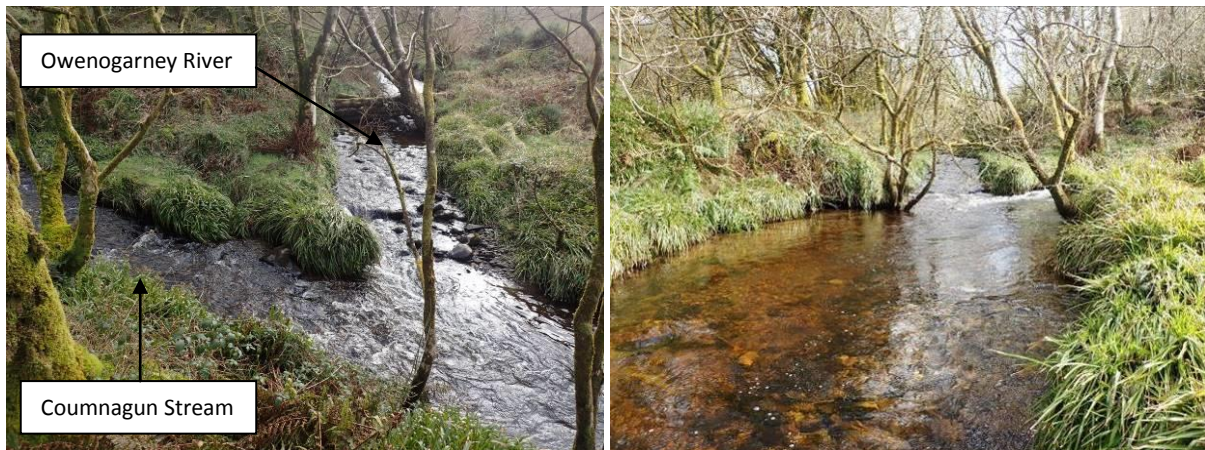
Plate 3 Coumnagun - Owenogarney confluence: notch stone weir on both watercourses to create plunge pool.
