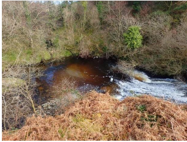
Plate 34 Some minor branch clearance at RHS of channel.
