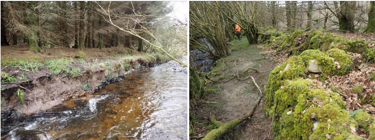
Plate 12 Bare banks along this reach with associated erosion of soils beyond the grip of conifer roots (left). Tunnelling effect on this reach along with past removal of large substrate from the channel has reduced instream heterogeneity and ecological value (right).
