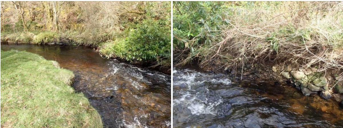
Plate 18 Remove rhododendron and install bank protection upstream of confluence with minor stream.
