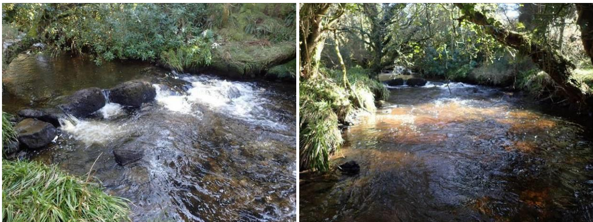
Plate 27 Incomplete boulder bar across the river: fill gap at LHS with a boulder(s) to develop a plunge pool. View from RHS bank (left), view upstream (right).
